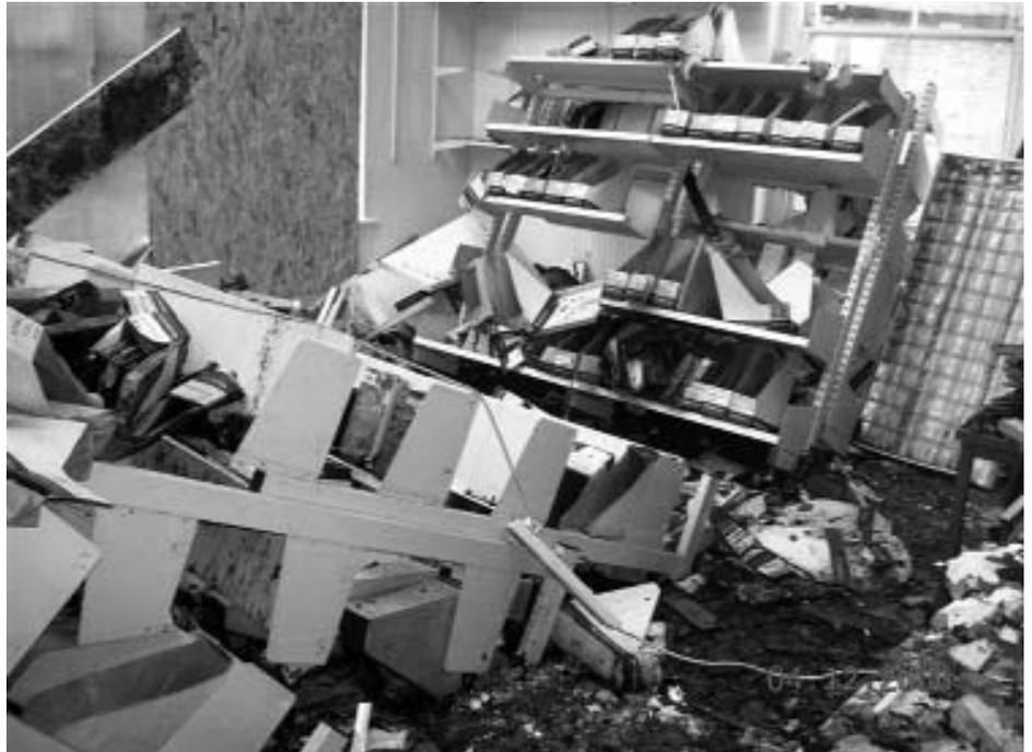
Burning beams and collapsing ceiling fell on to the shelving
